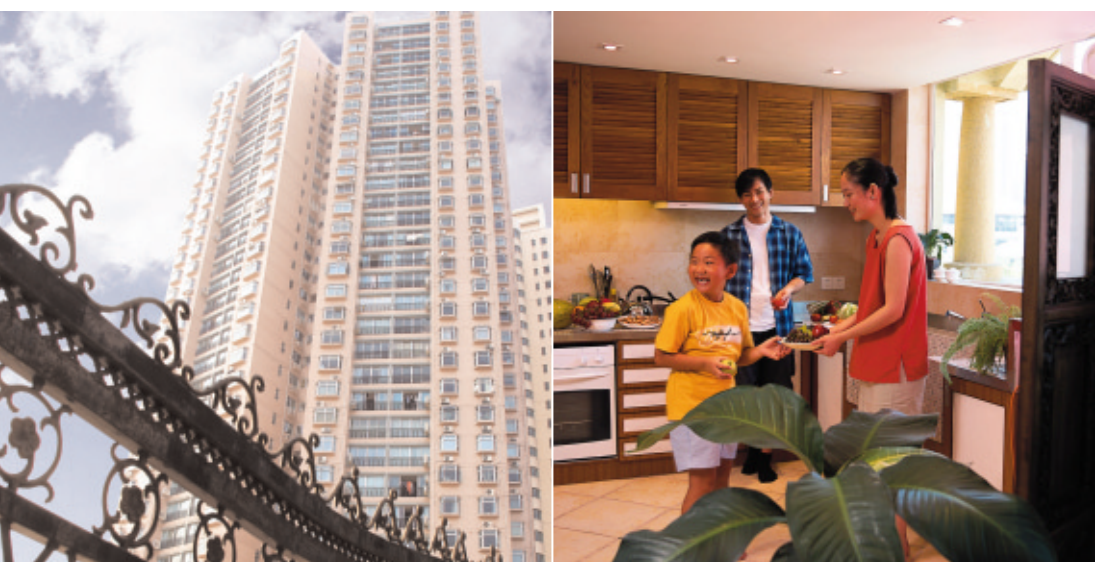
Far left, part of the residential portion of Shanghai Hong Kong New World Garden. Left, this spacious and well-designed kitchen is typical of the high-quality interiors at this development.
