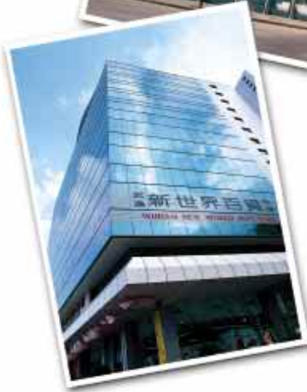
Annex building of Wuhan International Trade & Commerce Centre
