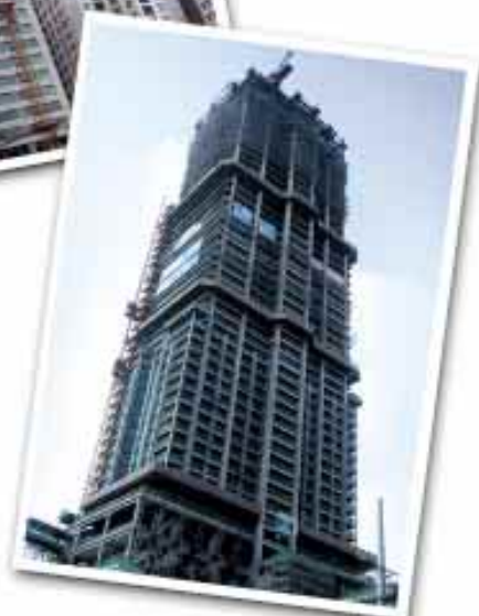
Hong Kong New World Tower
