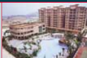
Completion of Guangzhou New World Eastern Garden Phase I
